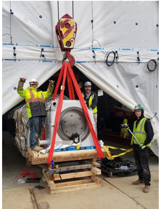
Millwrights Local 1121 working in Barnstable at Vineyard wind substation
