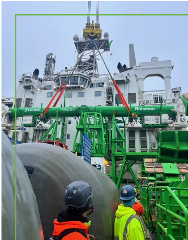
Pile Drivers and Divers Local 56
